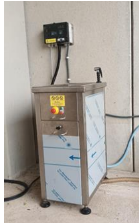
Figure 1: Electrolux brand commercial shredder installed in the Spanish EcoSite.
